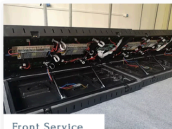
Front Service Cabinet
